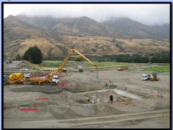
The weather has now settled down to long hot days which allows for good onsite progress. Foundations are being progressively poured in both the Hotel and Apartment buildings. Multiple activities are planned for March with structural steel arriving late in the month.
